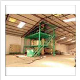
15 Tpd Cattle Feed Plant
